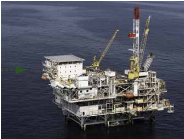
The petrochemical sector is just one industry which chooses Global pumps as it is leak-free and performs exceptionally well in critical areas
